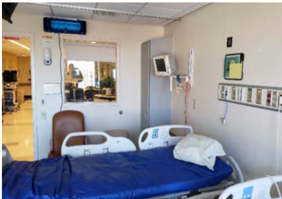
Figure 4. Upper room ultraviolet germicidal irradiation (UVGI)
